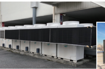
Heat-shield nets installed on outdoor units of air conditioners
