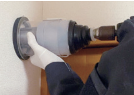
Work using a dust-dispersion-prevention cover
